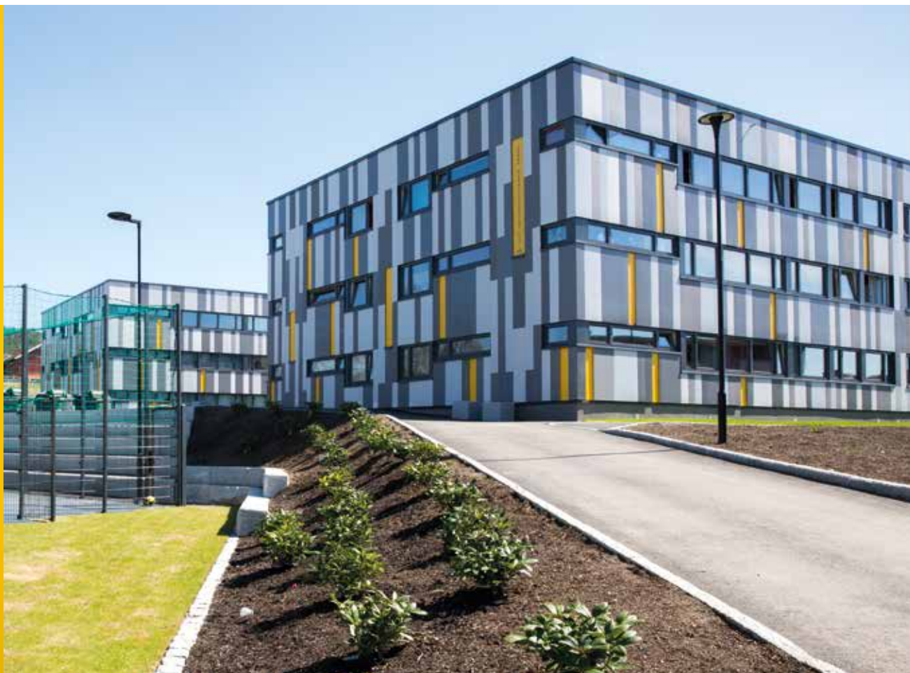
At Skullerud in Oslo, Boligbygg has renovated the housing complex into pleasant apartments with bright, exciting façades and green grounds.
